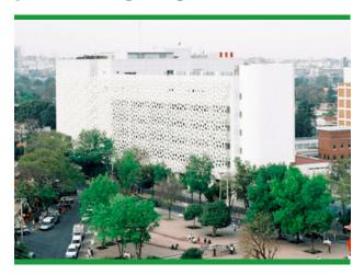
Completed in April 2013, the <u>Torre de Especialidades</u> building (part of the Mexico City hospital) absorbs and breaks down chemicals in the surrounding air. The construction features a layer of tiles painted with titanium dioxide, which reacts with UV light to break down pollution into less toxic chemicals such as CO2 and water. The Prosolve370e tiles were developed by Berlin-based design firm, Elegant Embellishments.
