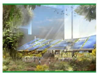
Opened in December 2012 in Hong Kong, the **Zero Carbon Building** produces more energy than it consumes. Using over 80 different green energy-saving technologies including photovoltaic solar panels, natural ventilation, micro-wind turbines and biodiesel fuel generators fed by used cooking oil, the building produces surplus energy of up to 99 megawatt hours per year, which is pumped back into Hong Kong's public power grid. It cost HKD 240 million to build.
